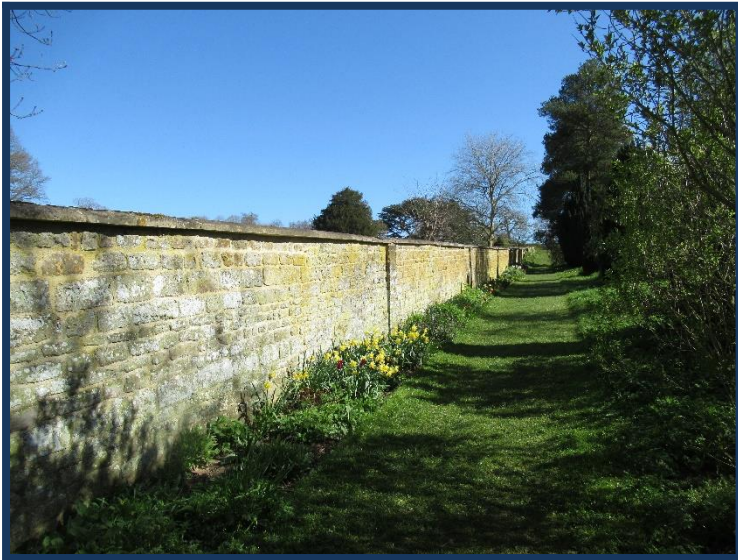
Figure 31: Listed walls within the grounds of Canons Ashby House
