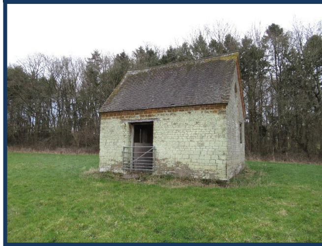
Figure 42: Barn northwest of Park Cottage
