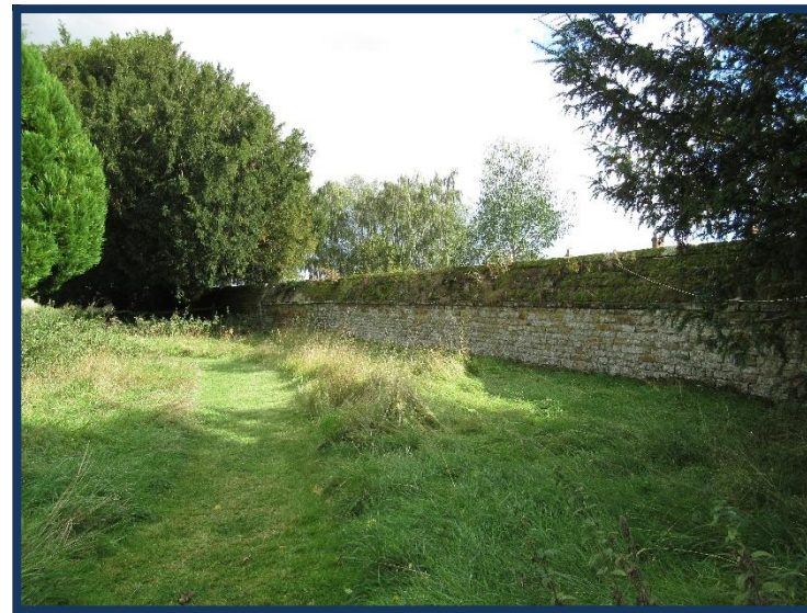
Figure 32: Wall of the 16 th century walled garden
